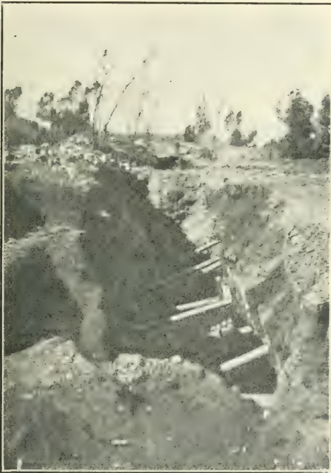
UNDERHAND STOPING ON THE MAIN REEF OUTCROP.
